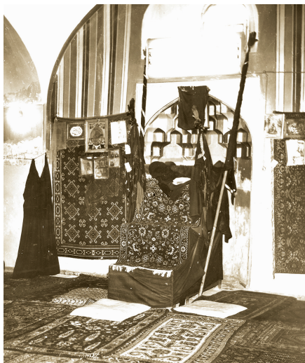
View of Demirbulag Mosque from inside destroyed by Armenian vandals. 1897.
